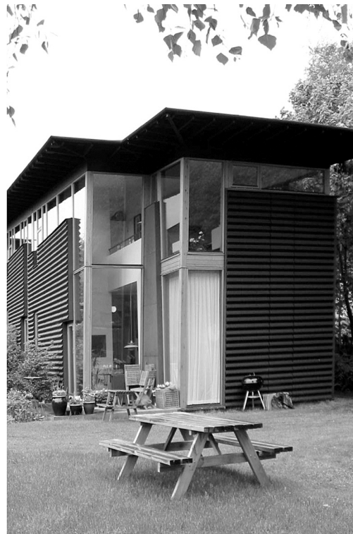
Fig. 4: One of the dwellings in the Søhusene complex included in the 1:1 tests
