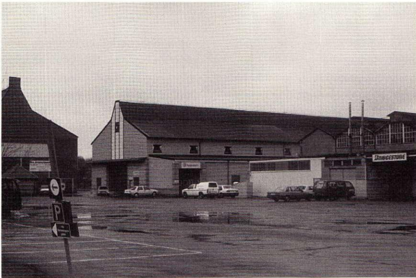
A small developer has renewed an old industrial estate, Grafiten, providing new office space at the entrance of the estate, as well as low cost, refurbished industrial space in less prominent locations. (Photo: Anders Törnqvist)
