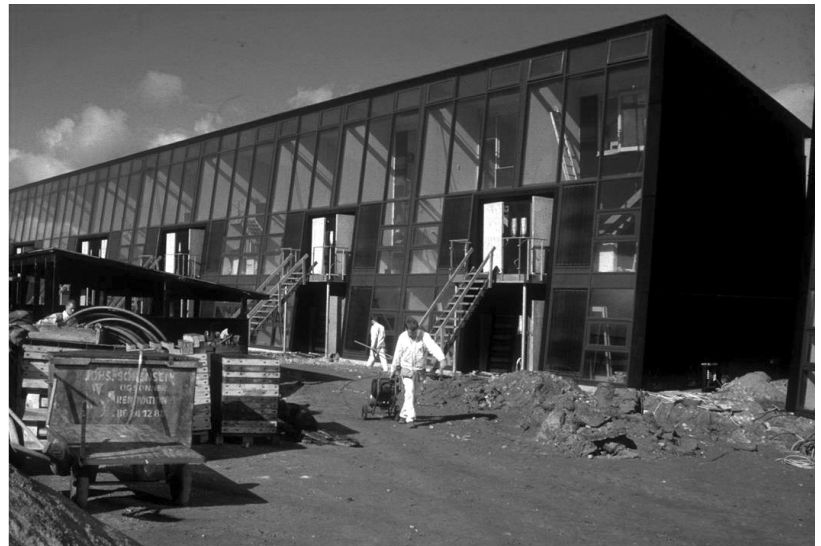
Picture 5: Vandkunsten (1998): Ecohouse 99. One-storey apartments with two-storey apartments on top. Solar rooms to the south.
