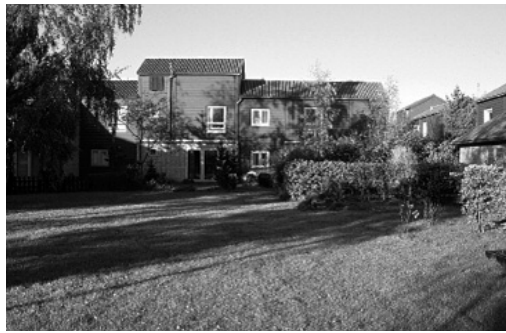
Picture 2: Vandkunsten (1978): Tinggaarden. Bearing concrete constructions with wooden cladding. Dense/low housing with very flexible house units and fine spatial potentials for user democracy.
