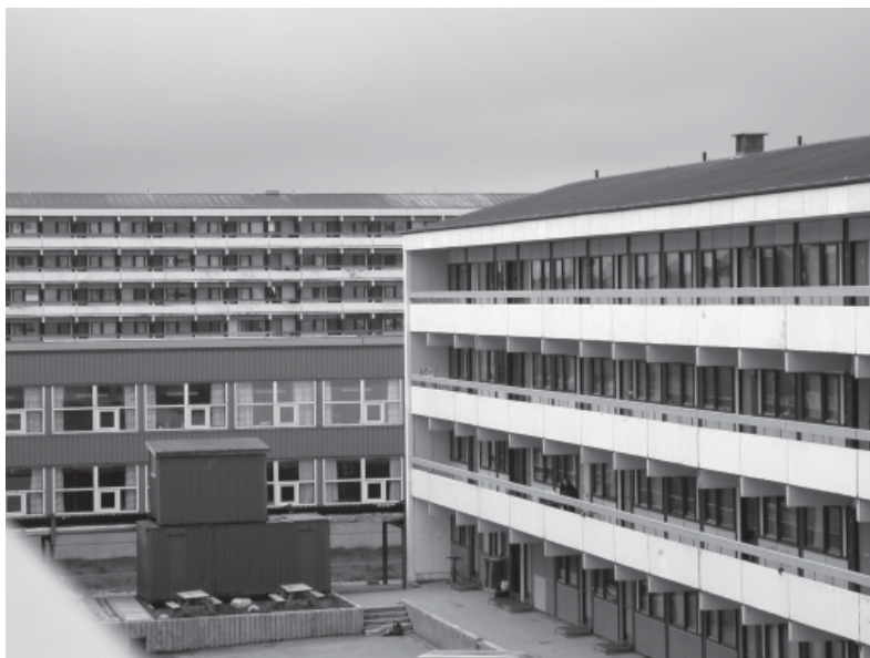
DSCN_8674 View of block 9, Uklusaq school and block P, Narsarsuaq housing project, Nuuk, Greenland. 17 August 2002 Narsarsuaq / Nuuk
