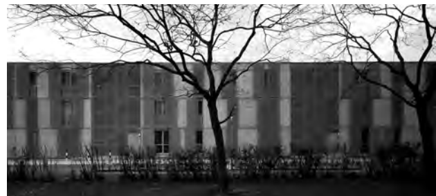
4: The façade of Strassgang
