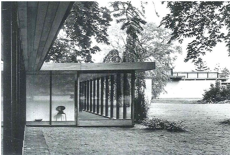
Figure 19 Historical picture of the North Wing of the Louisiana Museum.
