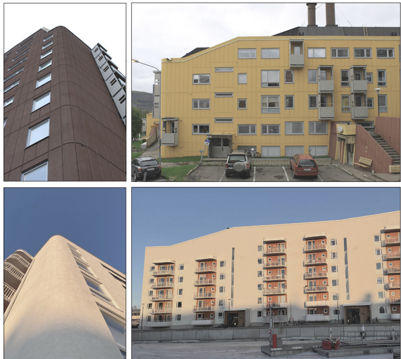
Figure 2: Between 1959 and 1965, architect Ralph Erskine designed the Ort drivaren neighbourhood in Kiruna, Sweden, featuring notable buildings like ‘Mullbänken’, ‘Snusdosan’, and ‘Spottkoppen’ (top row of photographs). The architecture exemplifies climate-responsive design suited for northern urban landscapes, a principle also seen in Luleå’s Southern Harbour, where buildings are designed to mitigate local winds (depicted below). Photos: the author
