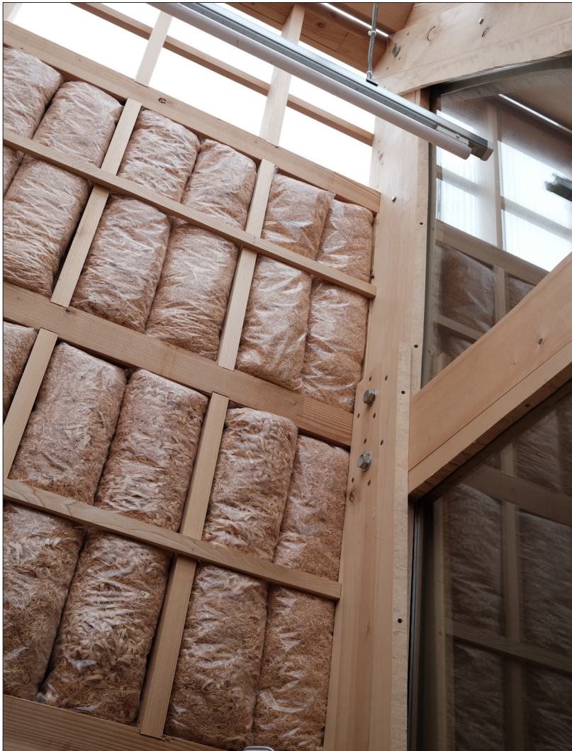
Figure 11: Morinha Office, sawdust insulation. Photo: the author
