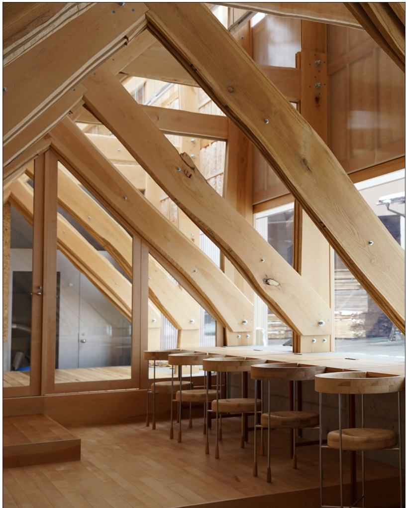
Figure 10: Morinha Office, wall and roof structure. Photo: Mooto Chiba, Tsubame Architects
