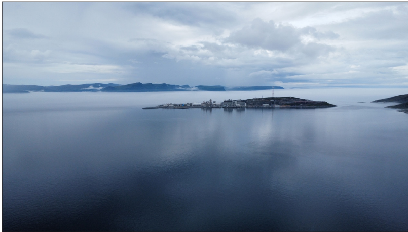
Figure 2: Melkøya island and the Hammerfest Liquefied Natural Gas plant. Source: Runa Johannessen
