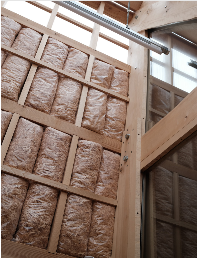
Figure 11: Morinha Office, sawdust insulation. Photo: the author
