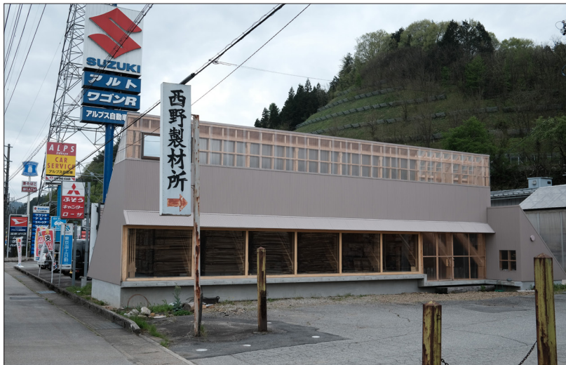
Figure 9: Morinha Office Building, Hida Furukawa, Tsubame Architects (2022). Photo: the author
