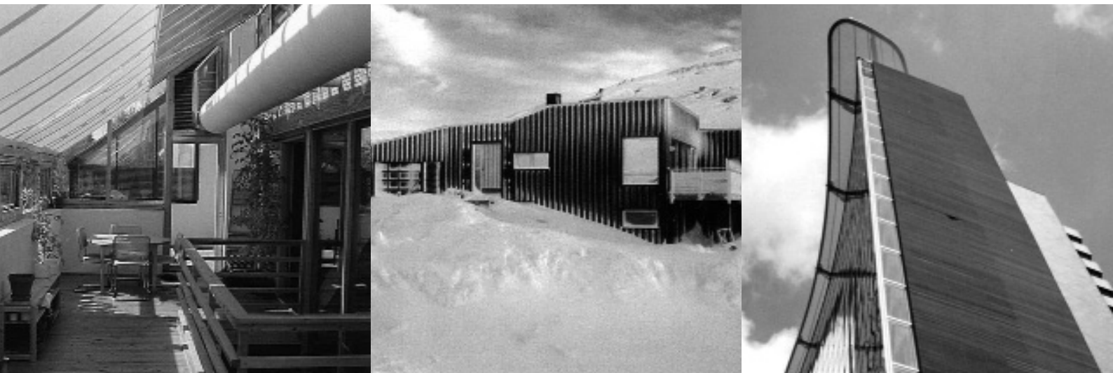
Figure 1: Measures for climate adaptations have strong implications for the overall design of buildings a) Norway: Sunroom in passive solar dwelling, Trondheim. Architect: Sintef/ Hestnes 1982. (Photo: F. Østmo) b) Norway: Wind adapted dwelling reduces snow drifts in Hammerfest. Architect: Børve/ Bjørge 1989 (Photo: O. B. Hansen) c) Germany: Wind roof facilitating natural ventilation at GSW Headquarters, Berlin. Architect: Sauerbruch Hutton Architects 1999 (Photo: T. Kleiven)
