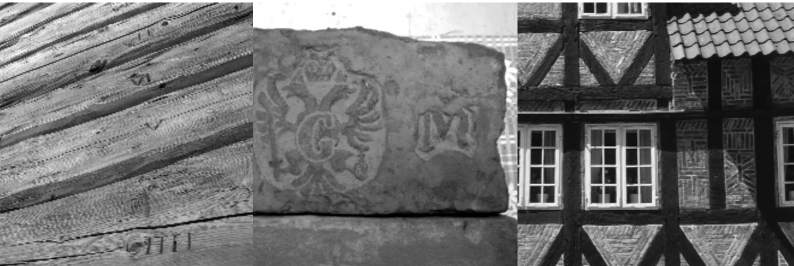
Figure 7: Useful information regarding salvageability can be carried along with the components as well as along with the architectural language a) Norway: Carved marks on traditional log construction defines the placement of each log in the system. (Photo: A. S. Nordby) b) Hungary: Old, reclaimed stamped bricks are popular as decorative reuse-objects. ( http://forum.index.hu ) c) Denmark: The readability of the architectural language gives access to information about material components and their reuse potentials. Half-timbered house in Holbæk. (Photo: F. Hakonsen)
