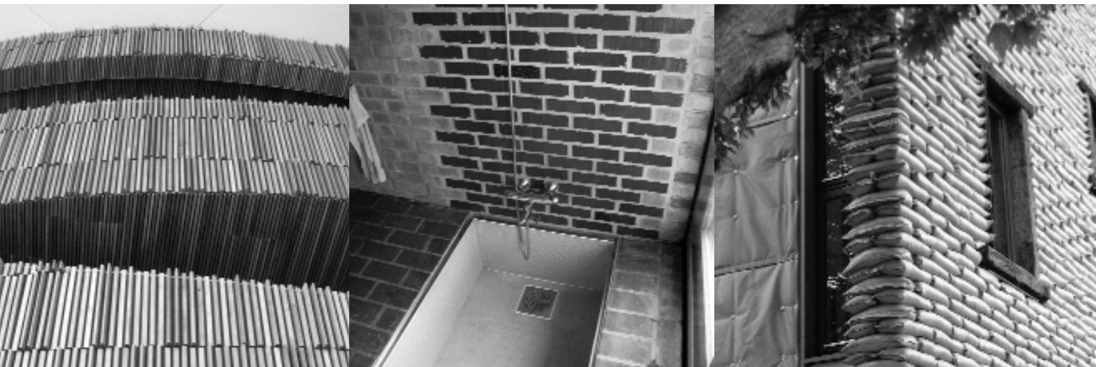
Figure 8: Physical properties of building components can meet constructional and environmental challenges, and at the same time substantiate tectonic relationships. a) Norway: Acoustic regulation in the grand foyer is facilitated by the use of panelling in oak that also add texture. Opera House, Oslo. Architect: Snøhetta. (Photo: A. S. Nordby) b) Norway: Moisture resistance and moisture capacity of bricks with different surface treatments are combined in a bathroom in Bærum. Architect: K. Hjeltnes. (Photo: A. S. Nordby) c) UK: Cloth cladding designed for a possible short-term life, and a more durable exterior skin of sand/ lime/ cement-bags are used in a combined office/ dwelling intended to change over time, London. Architect: S. Wigglesworth. (Photo: E. Wenn)
