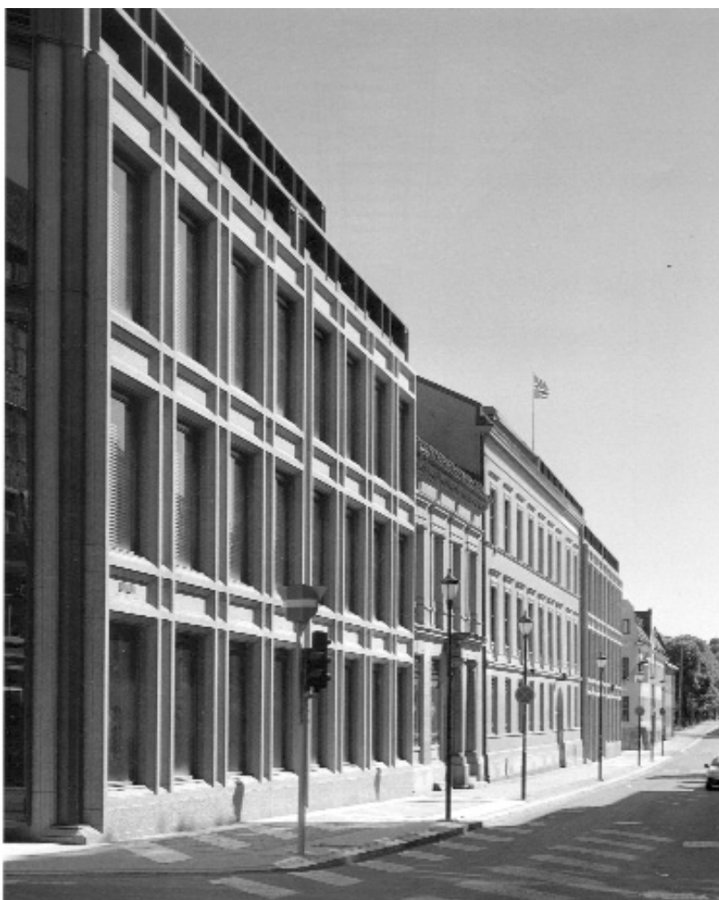
Fig. 11, Bank of Norway Head Office, façade as realized
