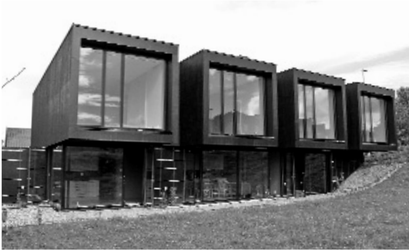
Garden and entrance side. (Photo: Bård Helland)
