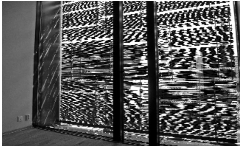
Entrance and window screen. (Photos: Bård Helland)
