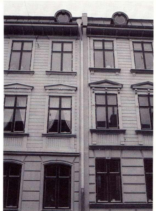
Typical façades in Gothenburg from the century turn, with the first floor built in brick and the upper two in wood (so called landshövdingehus ). These houses lie in Haga, which is now a conservation area. Photo: Solveig Schulz
