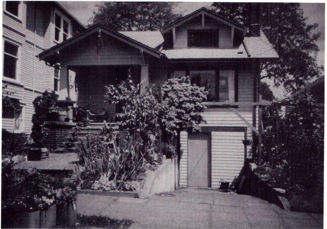
Photo of a narrow-and-deep bungalow with second unit inserted in the basement (see new door added).
