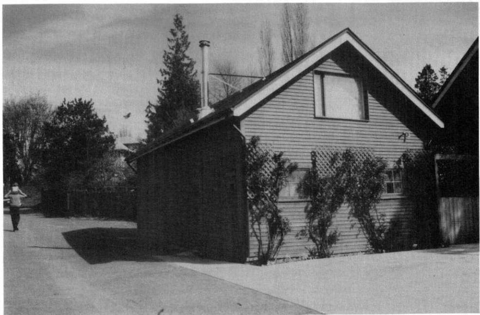
A garage apartment after conversion.
