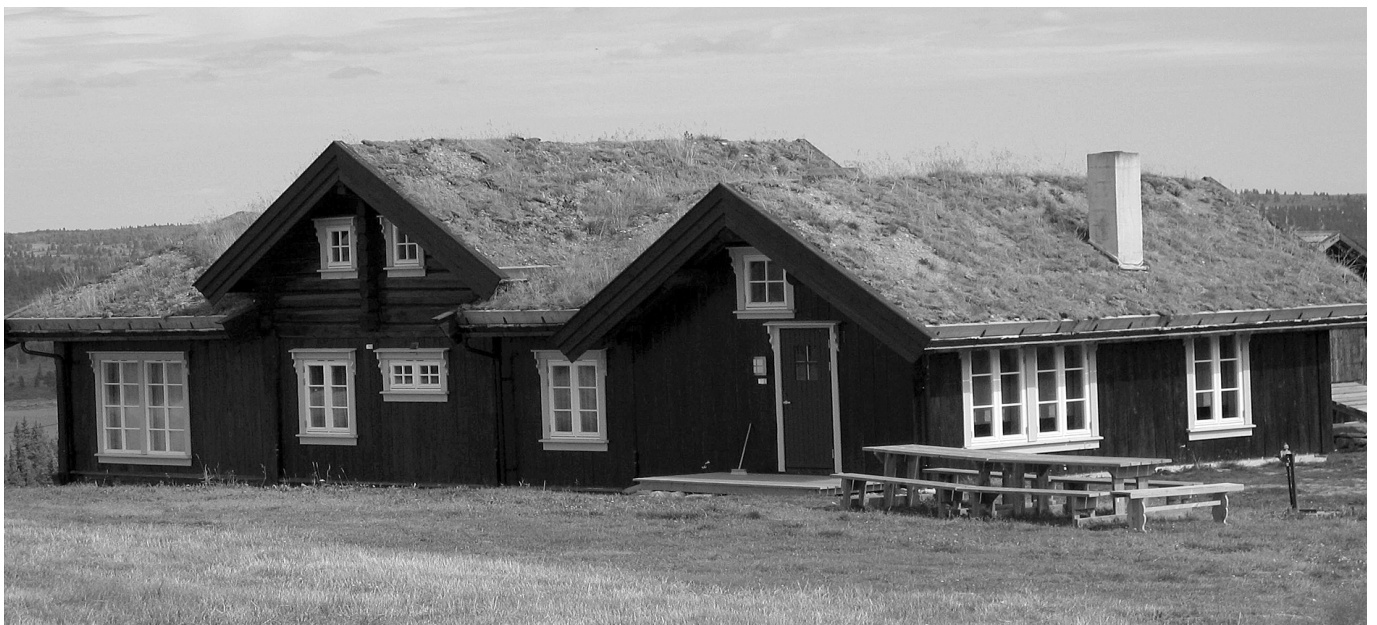
Figure 4: The extended stølsbu /cottage for hire. The old part is the right "wing" of the building with new windows, door roof and exterior panel. Photo: Authors
