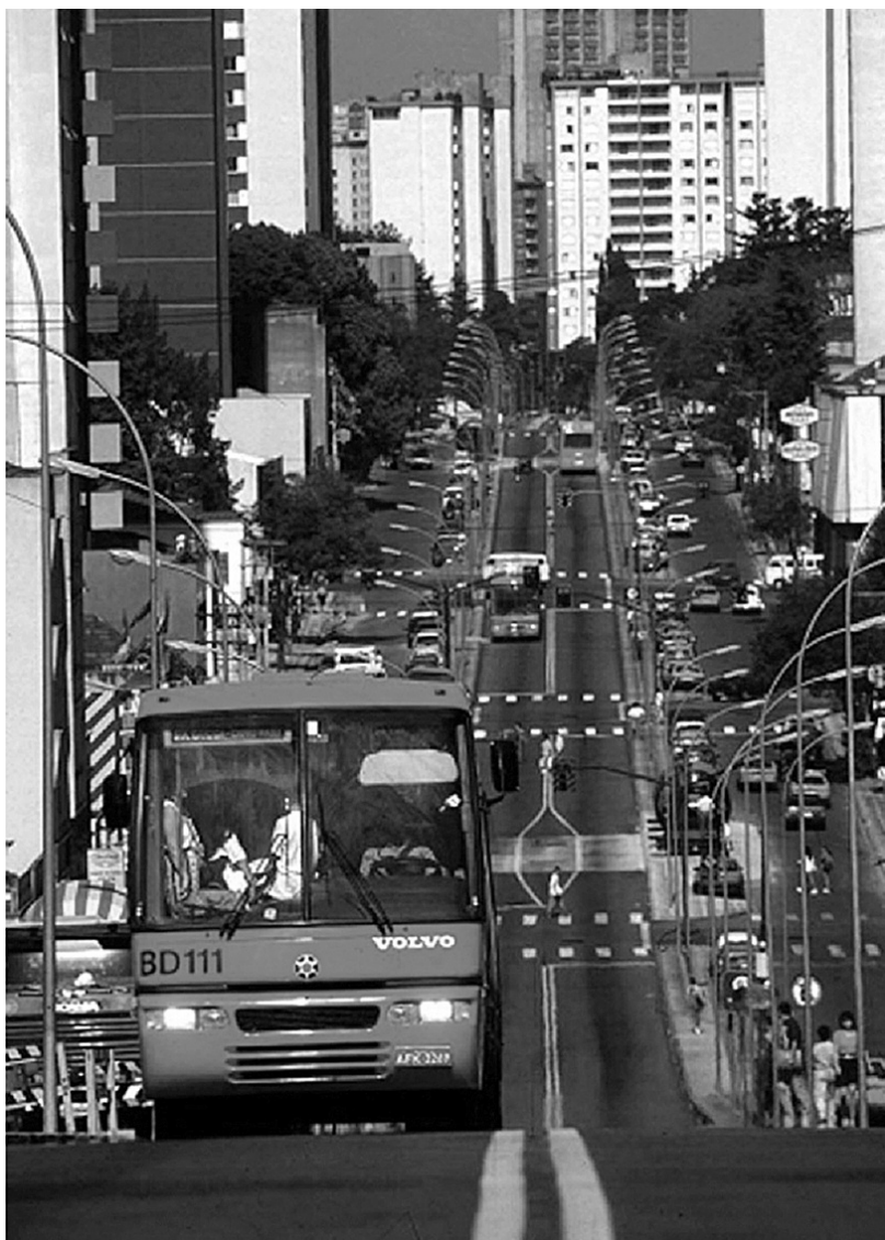
Figure 04: Curitiba BRT corridor with dedicated bus median lanes and high density along the corridor.
