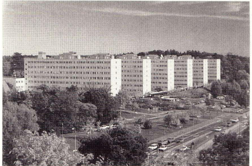
The South Building in Frescati, University of Stockholm
