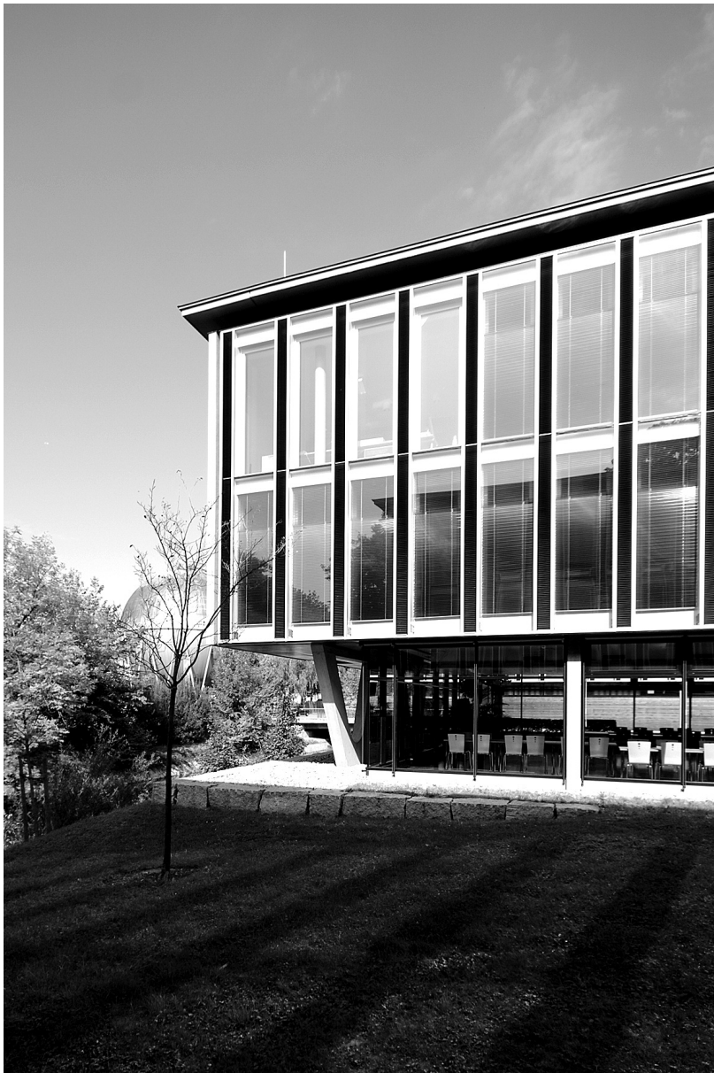
Figure 8: Badenova office building, Offenburg, Germany, by Lehmann Architects (2006). The use of phase change materials, natural daylighting and natural ventila- tion give a very low primary energy consumption without traditional HVAC solutions.
