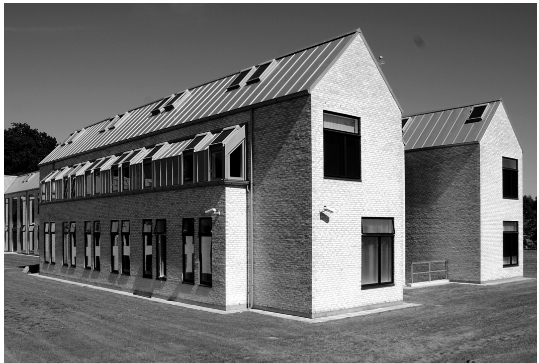
Figure 6 VKR Holdings headquarters, Hoersholm, Denmark, Hvidt & Mølgaard Architects (2007). Spatial proportioning creates high levels of well-distributed daylight. This provides a good working environment, low primary energy consumption, and no need for mechanical cooling.
