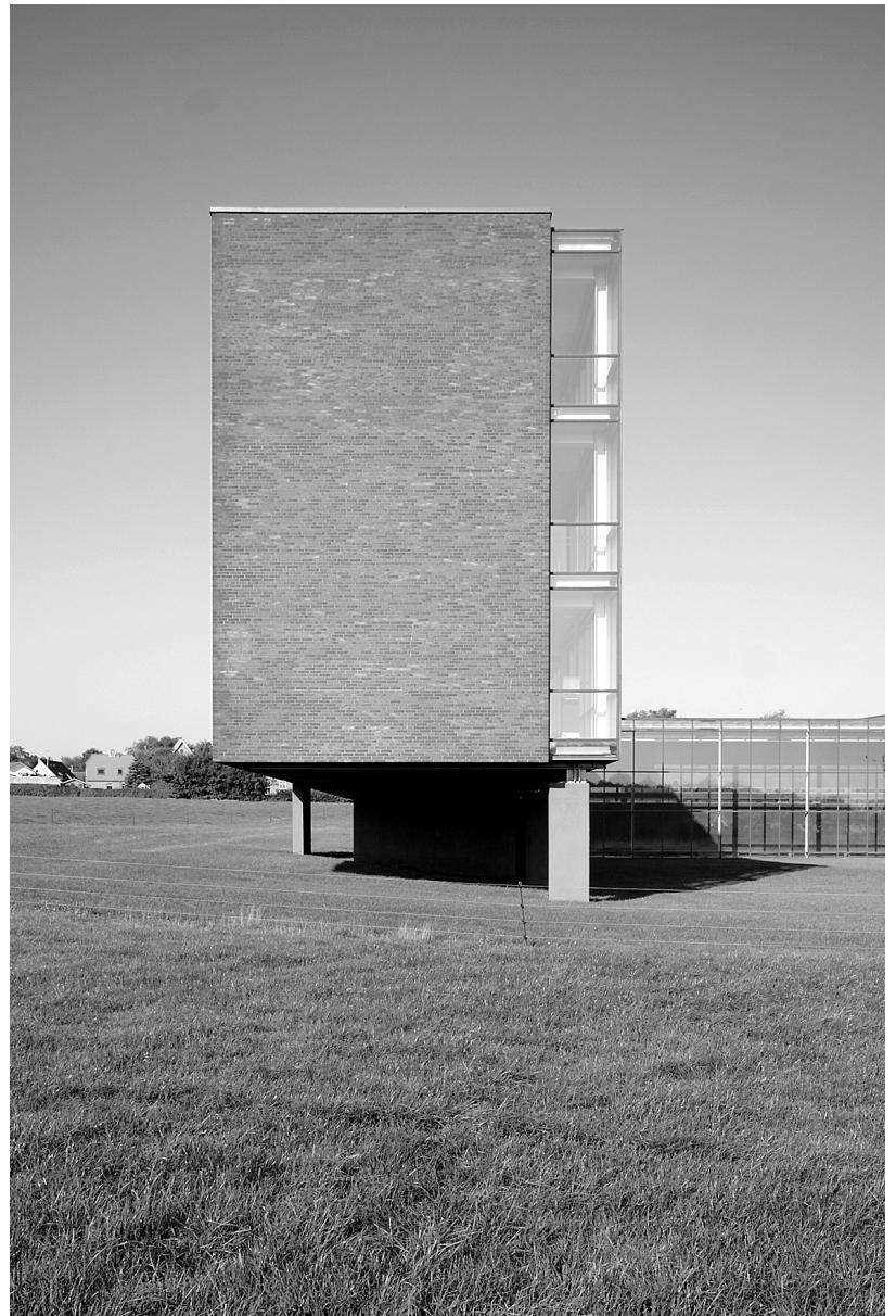
Figure 7: B&O headquarters, Struer, Denmark, KHR Architects (1998). The conscious use of northlight to create good visual comfort, minimise overheating, and utilise natural ventilation in the office spaces.
