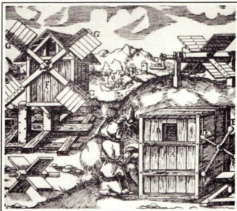
Figure 7. Ventilation of mine shafts.
