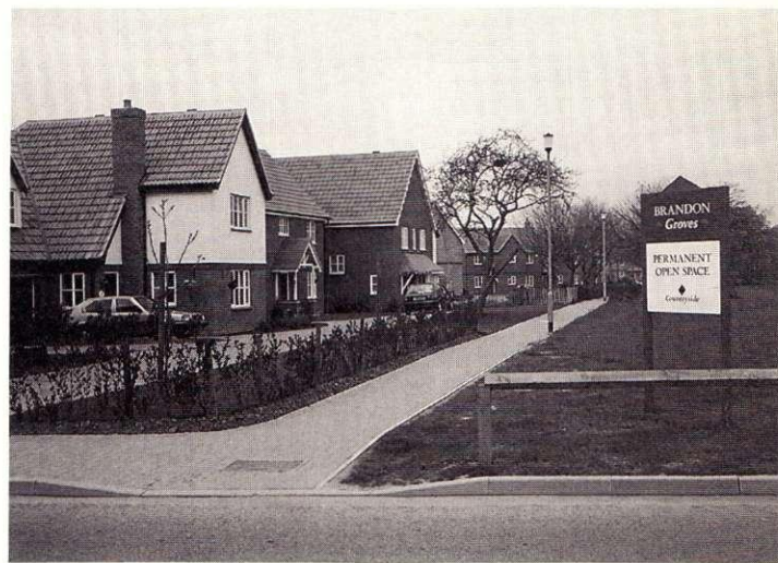
Plate 2. Neo-vernacular housing, South Ockendon
