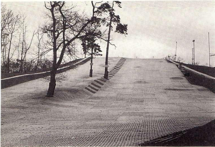
Plate 3. Built development associated with formal recreation: Brentwood Park
