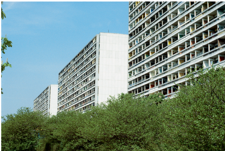
Figure 3 ‘The principle of equality’ was manifested in the buildings of the 1960s and 1970s. Homes were developed as standard types; a single standard type flat could be repeated again and again. The possibilities for adding special qualities to end-wall flats in the form of windows or balconies were not exploited. Similarly, the possibilities for designing the top-floor flats as penthouse flats with special qualities were rarely exploited. Photo: Claus Bech-Danielsen.
