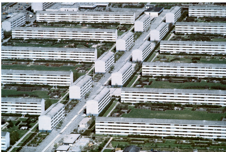
Figure 4 Buildings built along crane tracks. According to Jürgen Habermas, these are buildings developed with focus on an abstract system rather than on a concrete lifeworld. Photo: Claus Bech-Danielsen.
