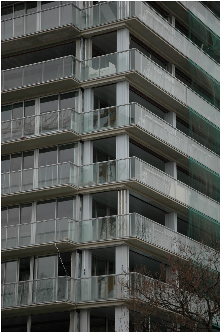
Figure 11 Tour Bois le Prêtre in Paris, renovated by Frederic Drout and Lacaton & Vasal. Photo: Claus Bech-Danielsen.
