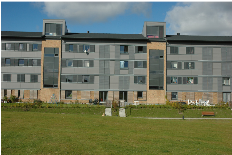
Figure 8 The balcony facades at Vejleåparken before (top) and after renovation (bot- tom). Photo: Claus Bech-Danielsen.
