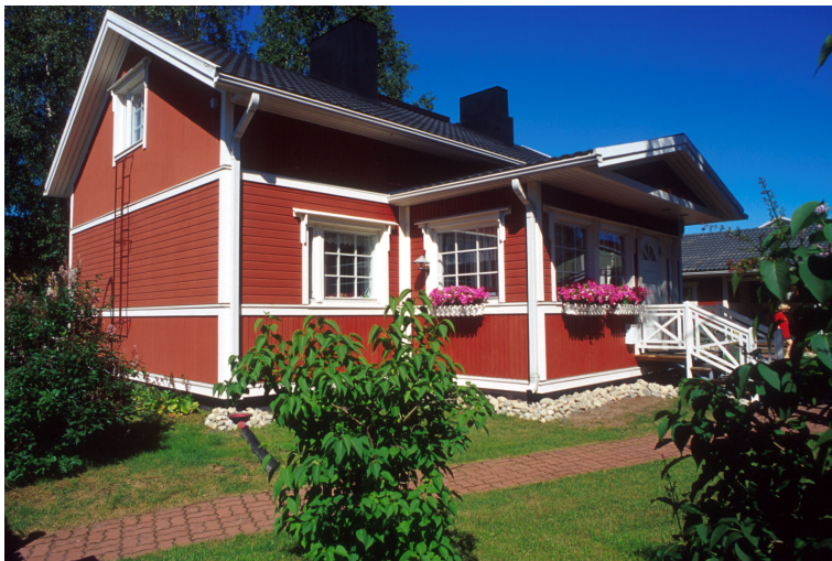
Figures 15 and 16 Many of the buildings has been refurbished and modernized completely from the outside as their modest appearance hasn't been appreciated. ANU SOIKKELI.
