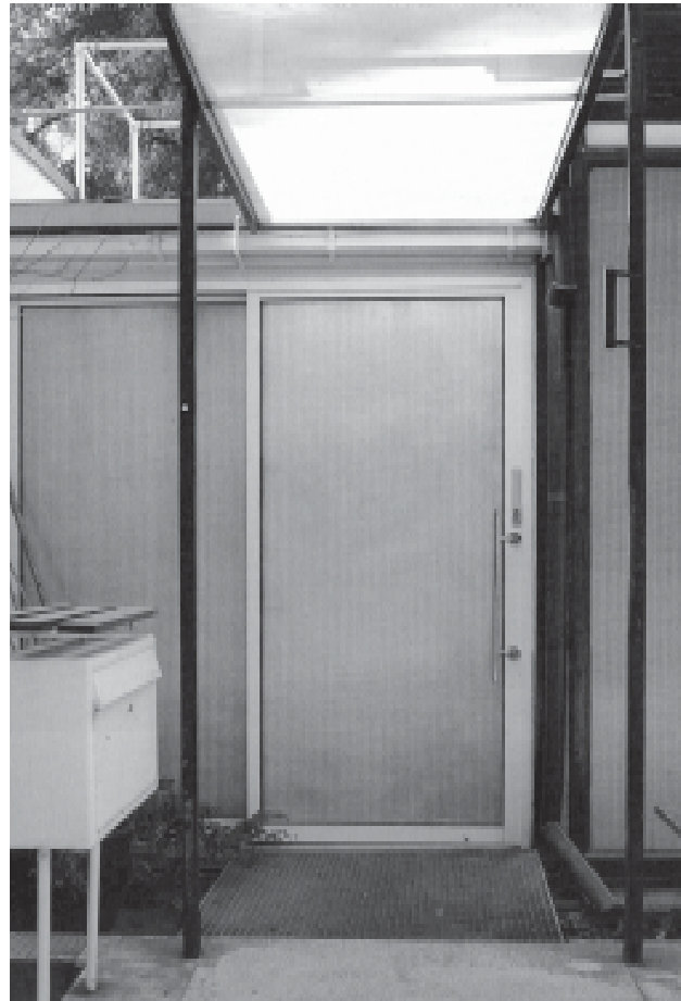
The Korsmo House, entrance
