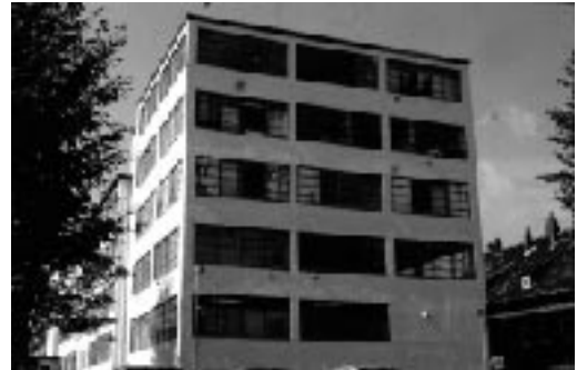
Storage building for Kappe & Co, Alfeld by Fred Forbat and Walter Gropius, drawn in 1922 and built in 1924.
