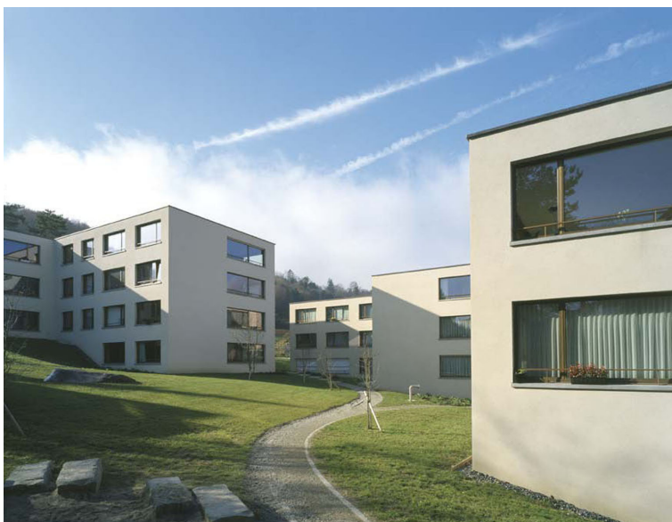
Figure 1. Bünzli & Courvoisier – Hagenbuchrain competition, exterior perspective of the competition and photo of the built project (source: Bünzli & Courvoisier, photo: © Hannes Henz)
