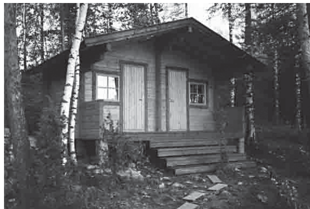
7. Model "Ranta-aitta 20" ["shoreline storehouse"], from Rantasalmen Huvilavalmistamo Korhonen Oy. An example of modern Finnish prefabricated cottages of Oivala's sauna type.
