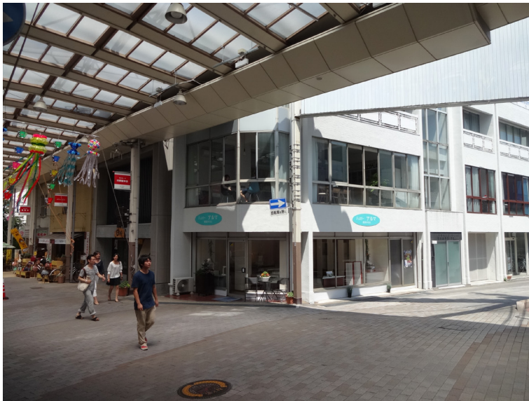
Fig 3 With the support of owners and volunteers, a three-story multi-tenant building located on a declining shopping street in central Maebashi that stood empty for already 15 years has been transformed into the student shared house Share Flat Babakkawa (2014). ©TOSHIAKI ISHIDA ARCHITECT & ASSOCIATES
