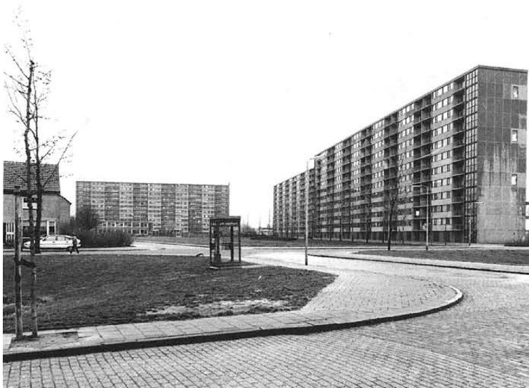
Figure 7 The original apartment blocks. The building on the right is called Schotteflat, presumably after the street named Schottestraat, (now named Johan Adriaen van de Perrestraat). These were the last buildings to be built with the BMB system in Zeeland (Coenen, Lentz and Prak, 1990, p.14). Reprinted from De Kopp is Eraf: Evaluatie van de aftopping van een flat in Middelburg, Michel Coenen, Gea Lentz and Niels Prak, 1990, p.9, with permission from IOS Press.
