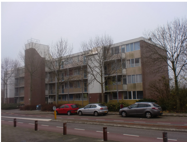
Figure 25 One of the three buildings made out of deconstructed panels, designed by architects van Pepper Jongepier, cf. Figures 7 and 22. The buildings are located in a quarter delimited by Vrijlandstraat, de Roozenburglaan and Buitenhovelaan streets.
