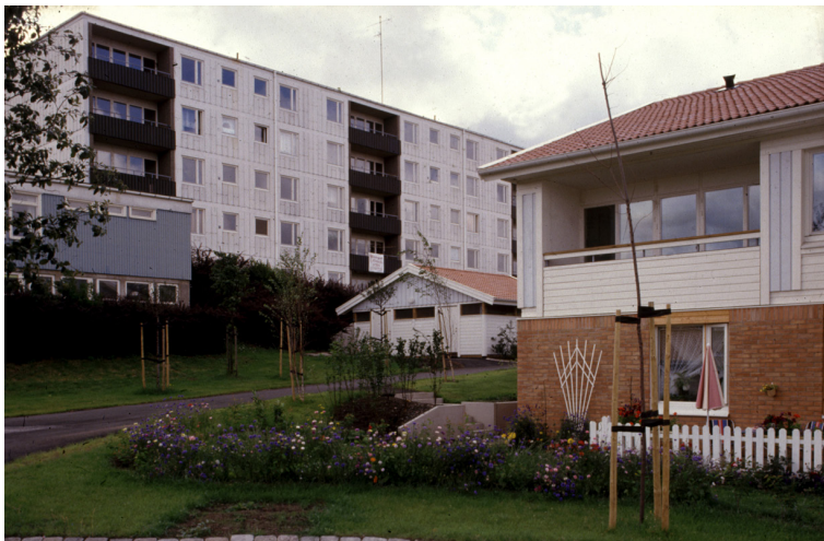
Figure 4 Buildings in Stjärnbyggsgatan street before the deconstruction (the block of flats on the left) and after it (the row-house on the right).
