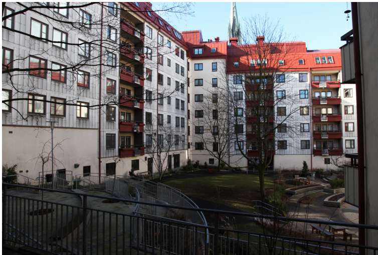
Figure 20 An apartment block on Prinsgatan/Plantagegatan streets, central Gothenburg, with reused panels in the courtyard facade. The street side has a brick facade to conform with the surroundings, and the slab was made anew. PHOTO: © CLAES CALDENBY.
