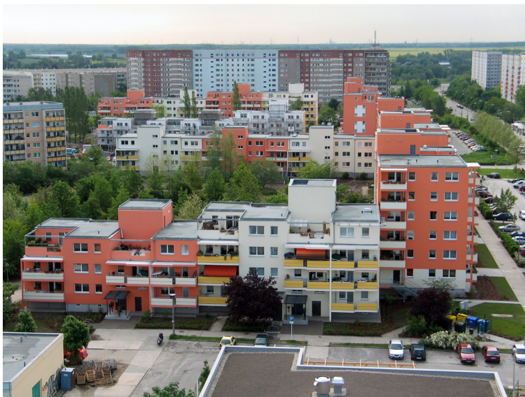
Figure 27 The finished project, now known as “Ahrensfelder Terrassen”, designed by architects Stephan Schüttauf and Michael Persike, cf. Figure 11. The final number of floors varies from 3 to 6. The transformation has been described as the largest urban regeneration project in Berlin, the volume of which is best described by the numbers of flats before (1,689) and after (447); the number of different types of flat was increased from 10 to 39 (Friedrich, 2015).
