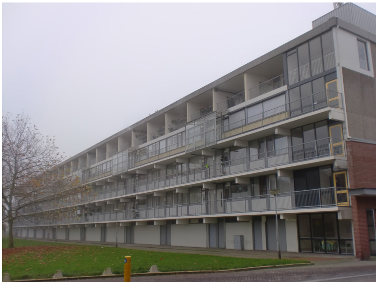
Figure 22 The deconstructed 5-floor Schotteflat, cf. Figure 7.
