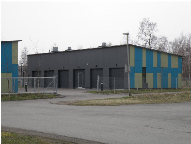
Figure 37 Garage for maintenance vehicles made out of the reused panels.
