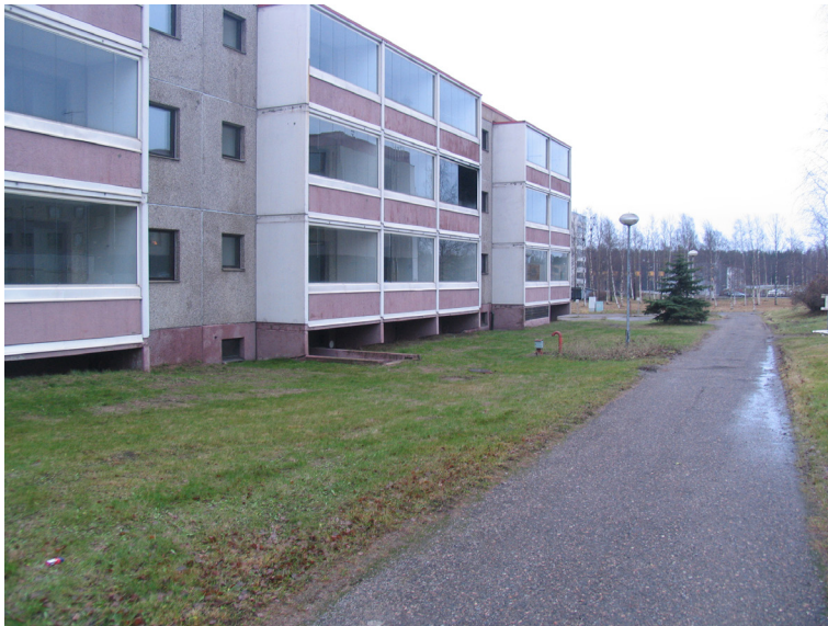
Figure 13 A 3-floor slab block in Jousikatu street.
