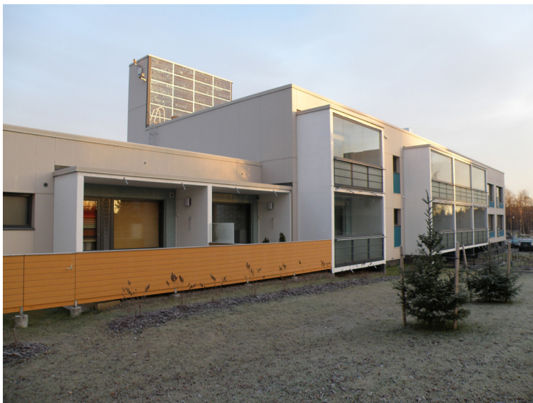
Figure 32 A slab block after deconstruction and refurbishment, designed by architects Harri Hagan and Petri Kontukoski, cf. Figure 13. The tower for solar panels is a new timber-framed structure.
