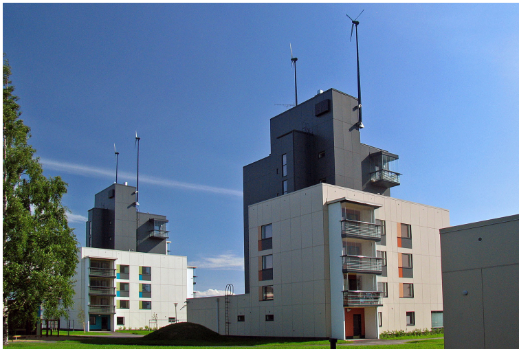
Figure 34 Point blocks after deconstruction and renovation, cf. Figure 15. When asked where the project failed, the housing company representative mentions the wind turbines; they have since been removed because they were constantly out of service.
