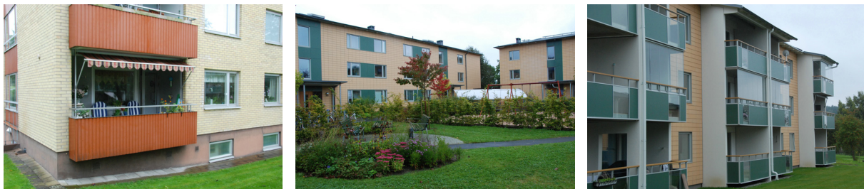
Figure 3 Case C before the renovation (left) and after (middle and right), showing the final design of the balconies.
