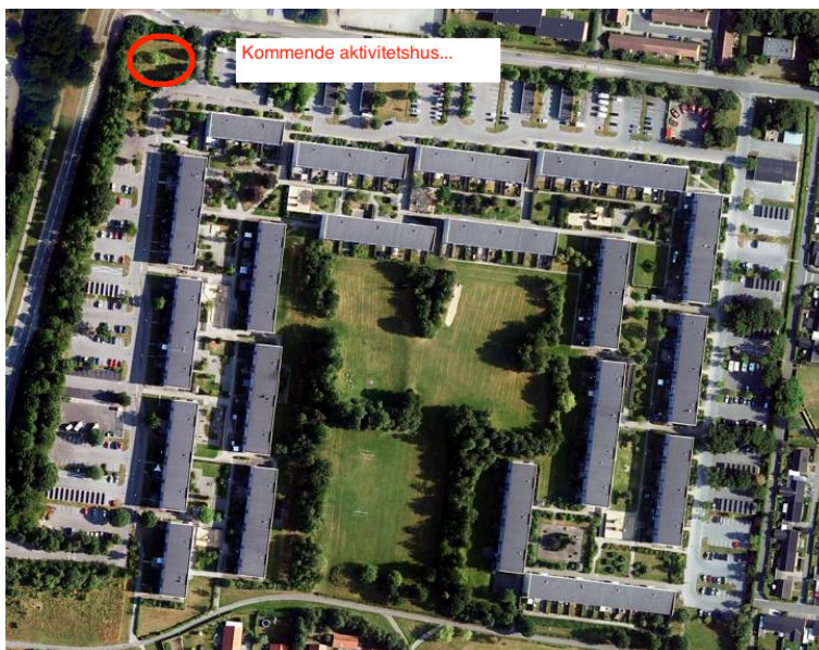
Figure 6 Situation plan, Houkærvenget with its identical building blocks in a horseshoe formation. The graphic, red spots points to the location of the new planned common activity house.
