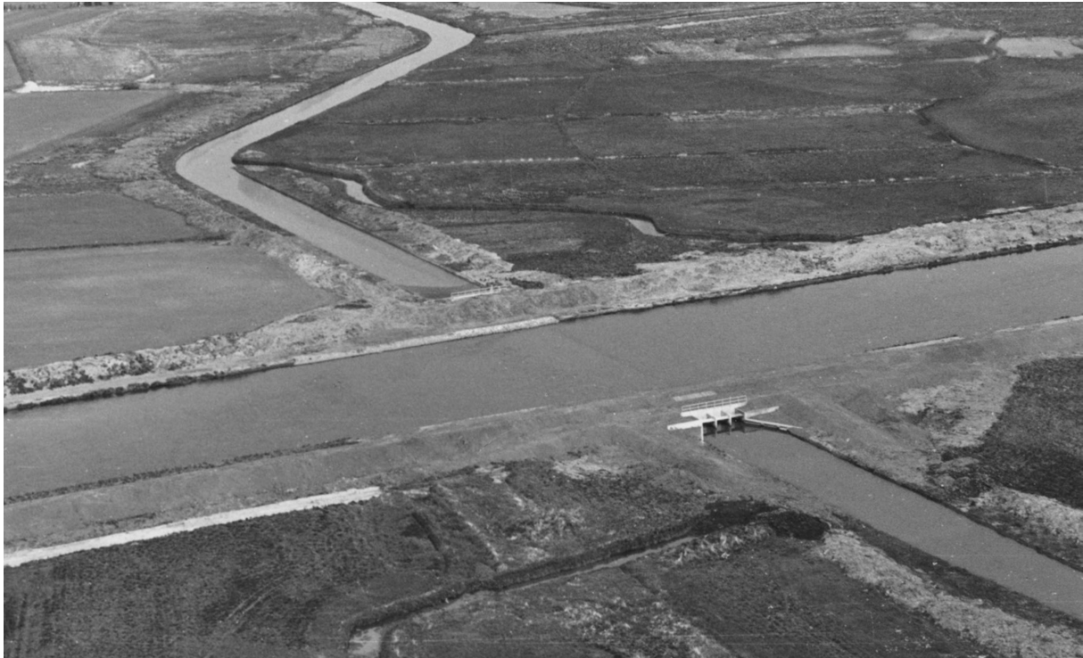
Figure 2 Water crossing. Source: Heath Society (Hedeselskabet) (1965). This aerial photo shows part of the extensive drainage system that was constructed as part of the ambitious land reclamation project in the Skjern River Delta. In total, 26 kilometres of the meandering river were converted into 19 kilometres of embanked canal, and 3,900 hectares of meadow and wetland became arable land. This highly engineered landscape also featured a "water crossing" where the Gæner River was directed under the Skjern River. Today most traces of these remarkable landscape features have disappeared, and in the process of nature restoration, curved lines have replaced straight lines.
