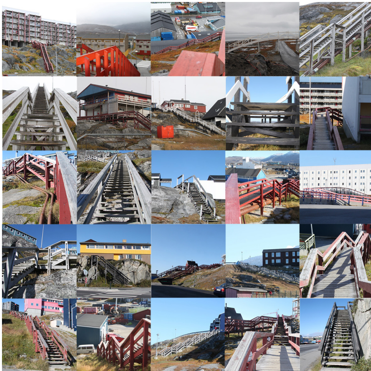
Figure 8 Modularity: a timber public stair design is repeated throughout Greenland, simplifying and streamlining this transport infrastructure (Carruth, 2015).
