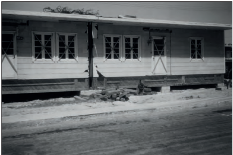
Figure 3. A Swedish duplex being prepared for relocating. Photographer unknown, Courtesy of King Abdulaziz Foundation for Research and Archives (Darrah).
