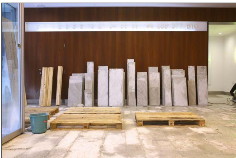
Figures 1–2. Rotor DC crew dismantling floor slabs in Carrara marble in the lobby of an office building in the European district of Brussels. Source: Rotor.
