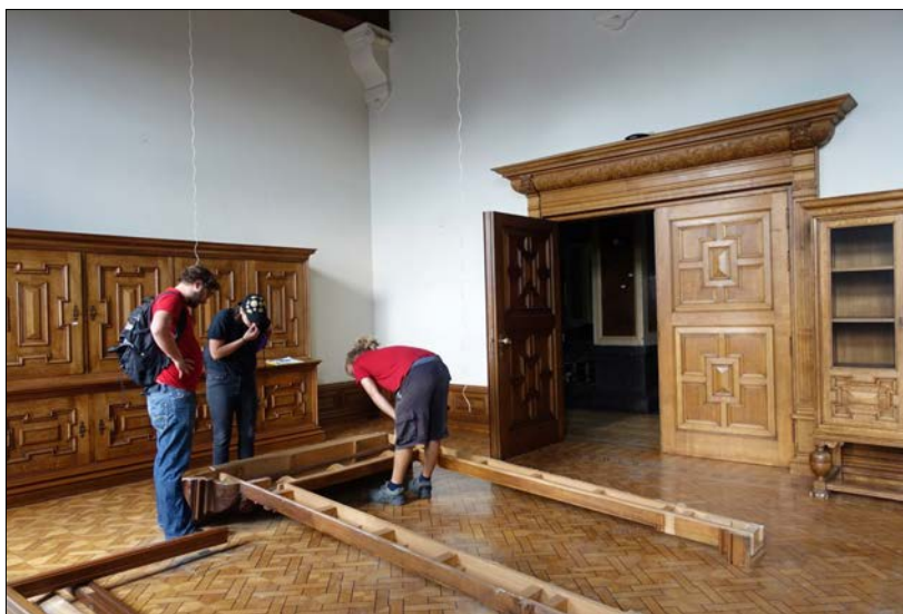
Figures 6–8. Deconstructing sculpted oak features during the remodelling of the interiors of Antwerp City Hall in 2017. Source: Rotor.
