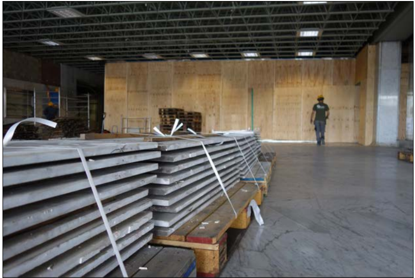
Figures 13–16. Dismantling of wall and floor panels in marble in the Brussels North Station. This part of the station was designed in the 1970s and is now being thoroughly remodelled. The panels, a particular variety of Carrara marble called Arabescato, are carefully stacked for transport. Source: Rotor.
