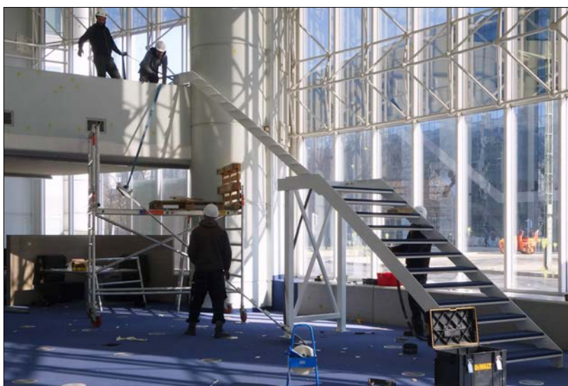
Figures 9–12. Rotor DC carefully dismantled the staircase in the lobby of the Boudewijn building in Brussels. Originally constructed in 1990, the government building is slated for demolition. Source: Rotor.
